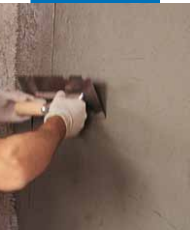
Applying Planitop 540 with a metal trowel
