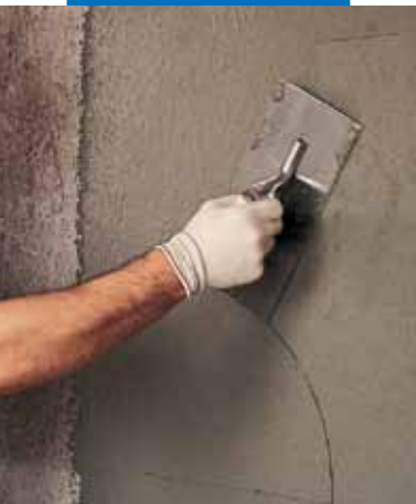
Smoothing the Planitop 540 surface with a metal trowel
