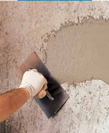
Applying Planitop 540 with a metal trowel
