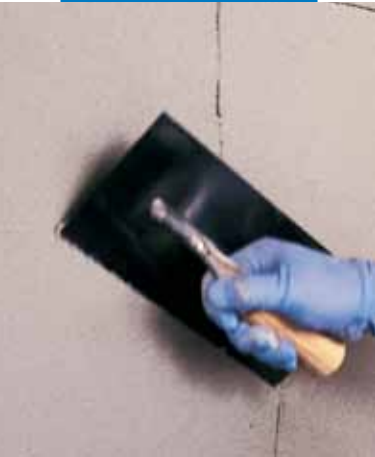
Applying Planitop 560 with a metal trowel
