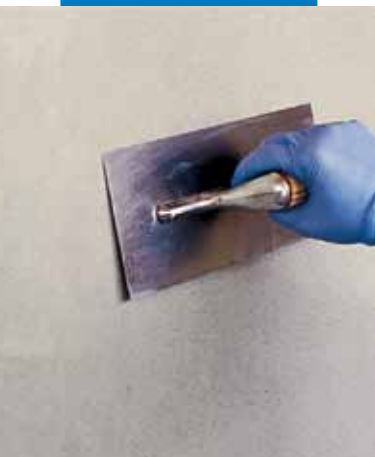
Smoothing Planitop 560 surface with a metal trowel
