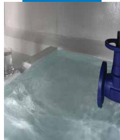
Filling the tank after Mapecoat DW 25 has completely hardened
