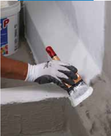
Application by brush of Triblock P on damp substrate
