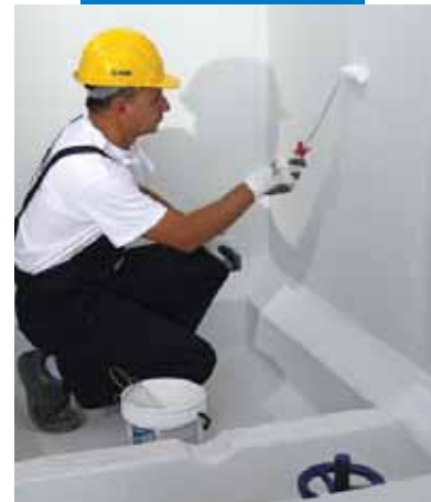
Application of Triblock P by roller
