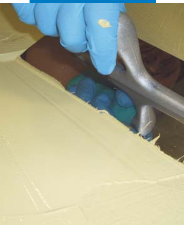
Application of Mapecolor Paste using a smooth trowel
