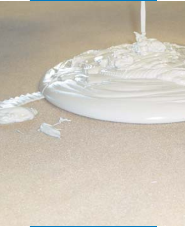
Mapecolor Paste poured on the substrate immediately after mixing
