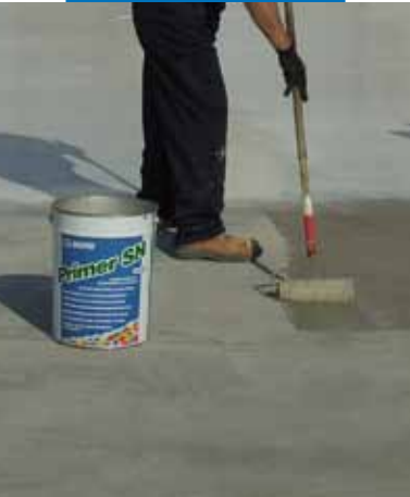
Application of Primer SN on a concrete floor slab with a roller
