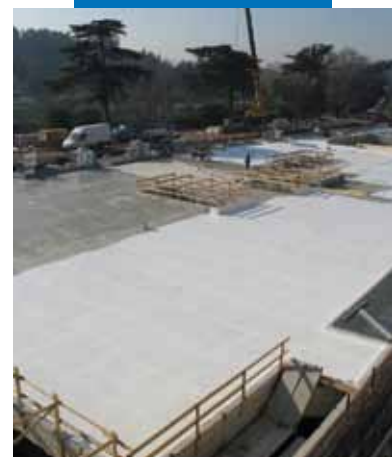
Covering of an underground car-park waterproofed with Purtop 600
