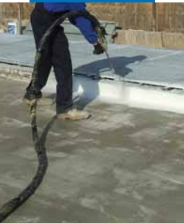
Application of Purtop 600 on a vertical overlap by spray
