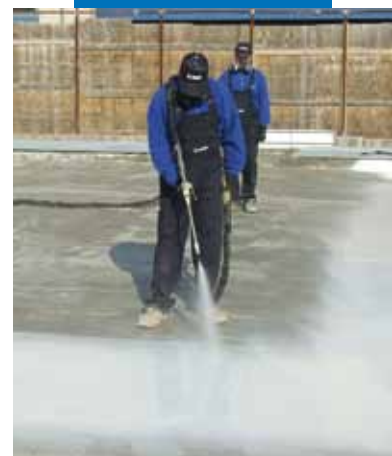
Application of Purtop 600 on a flat roof by spray
