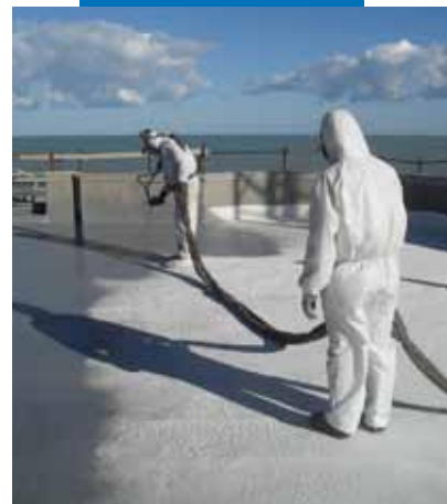
Application of Purtop 400 M over Triblock P
