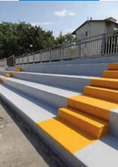
Spectator terraces waterproofed with Purtop 400 M coated with Mapefloor Finish 55
