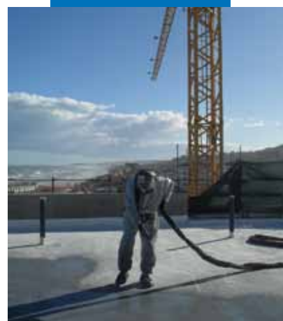
Application of Purtop 400 M over Triblock P
