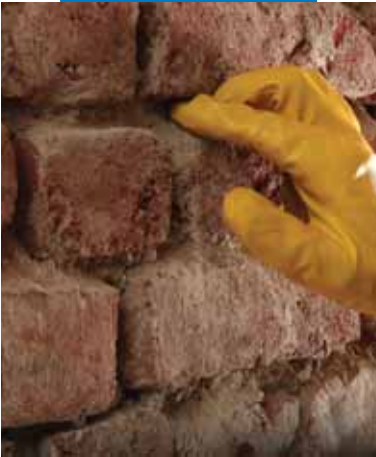
Consolidating the substrate
