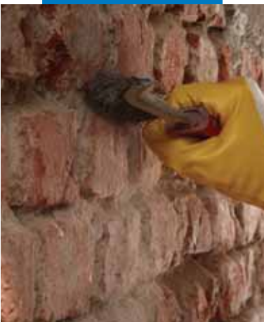
Preparing the substrate
