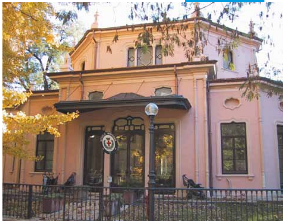
An example of an application of Silexcolor Tonachino . Nursery School - Porta Venezia Gardens (Milan) - Italy
