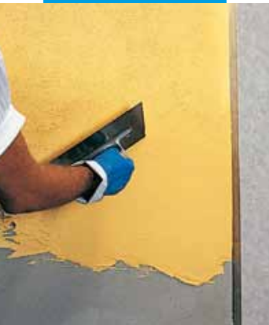
Applying Silexcolor Tonachino with a trowel
