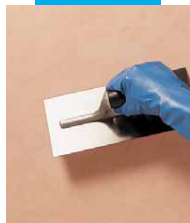
"Encausto" effect: glossing of Silexcolor Marmorino with edge of a stainless steel float
