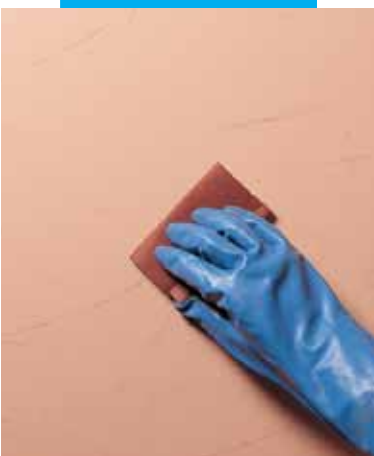
Classic effect: sand-papering of the first coat of Silexcolor Marmorino with a fine grained abrasive sand paper
