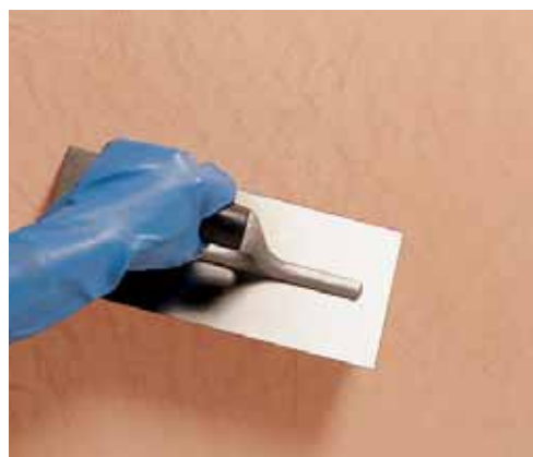
"Veneziano" effect: glossing of Silexcolor Marmorino with edge of a stainless steel float
