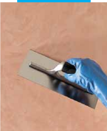
Classic effect: glossing of Silexcolor Marmorino with edge of a stainless steel float
