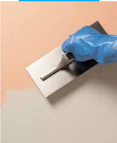
Classic effect: application of first coat of Silexcolor Marmorino with a stainless steel trowel
