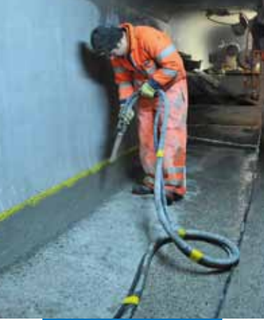
Application of Mapefinish HD by spray
