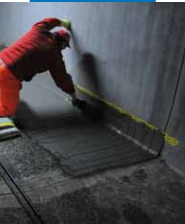
Smoothing over Mapefinish HD with a metal spatula
