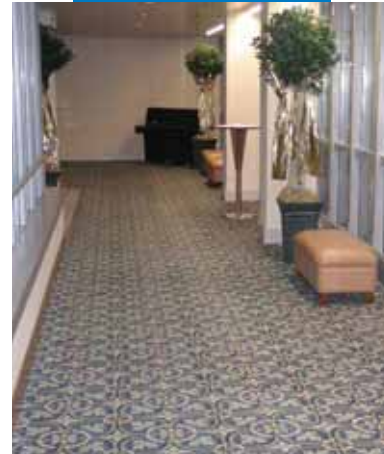
Carpet laid on a hotel corridor after levelling with Ultraplan Eco - Hotel Renaissance - Austria
