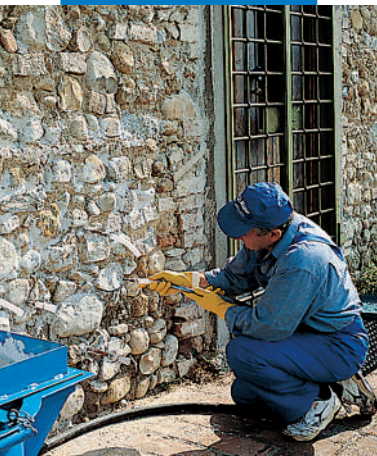
Consolidating injection with Mape-Antique I
