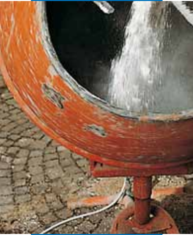
Mixing mortar on site with locally-sourced aggregates
