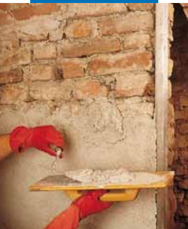
Application of de-humidifying render mix on site
