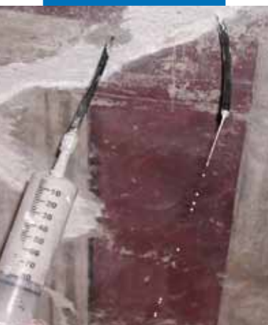
Injecting Mape-Antique F21 into frescoed wall
