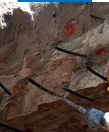
Injecting Mape-Antique F21 into stone masonry
