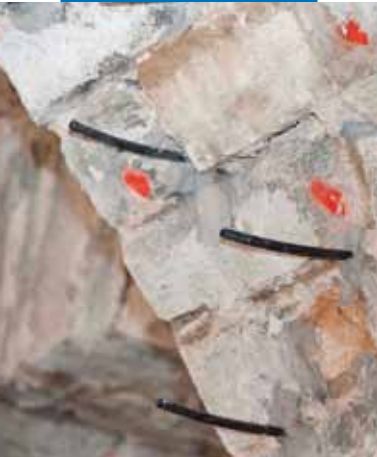
Detailed view of flow the injection tubes are fastened in place
