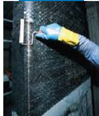
Applying a second coat of Mapewrap 31
