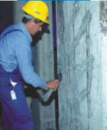
Preparing the substrate
