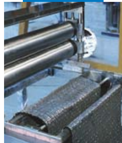
Impregnating Mapewrap C with a machine
