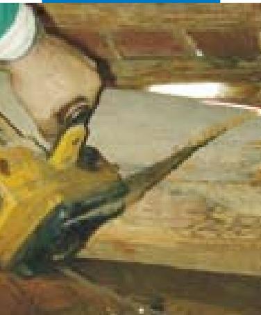
Sawing a beam
