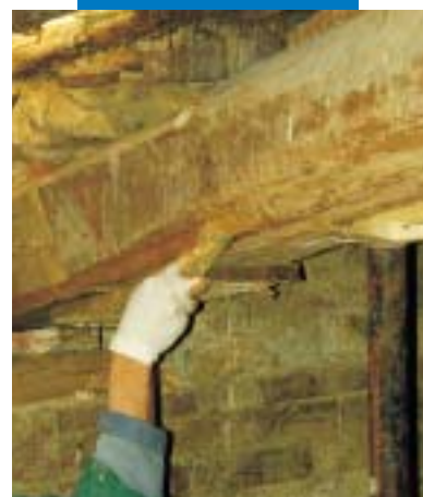
Applying Mapewood Paste 140
