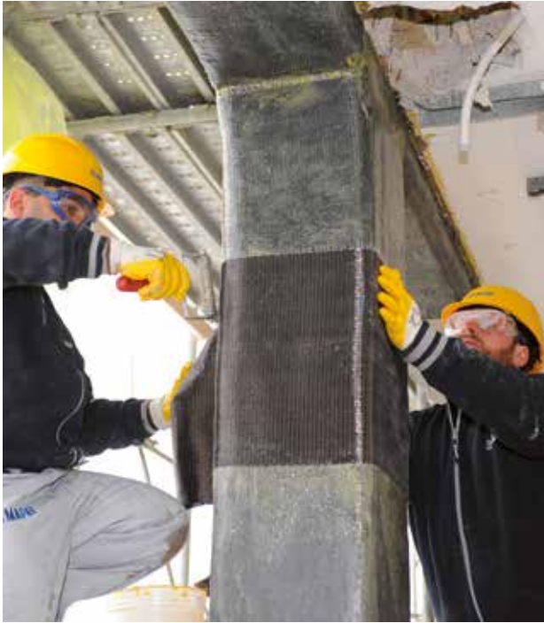
Strengthening of a beam-pillar joint with MAPEWRAP C SYSTEM – i Guzzini
