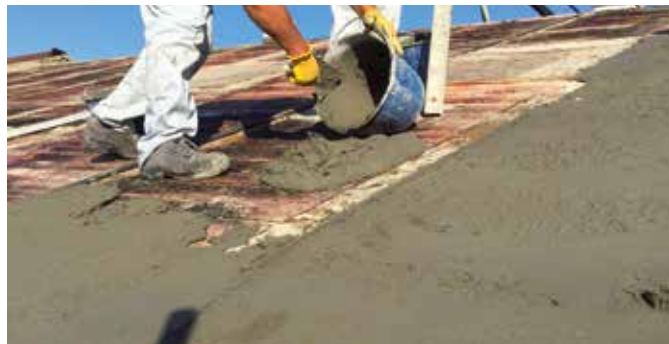
Strengthening of a sloping roof
