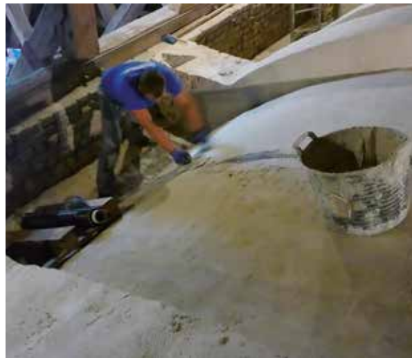
Strengthening package for the extrados of a masonry vault
