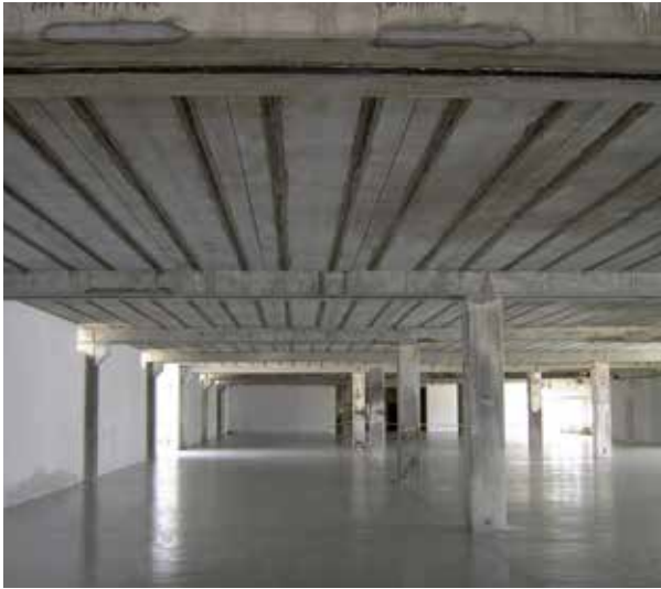
Flexural strengthening of beams and a floor with CARBOPLATE SYSTEM
