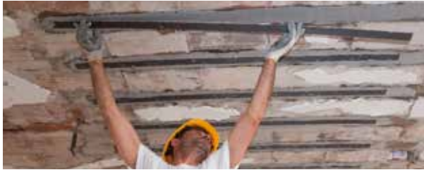
Application of CARBOPLATE SYSTEM on brick-cement floor joists
