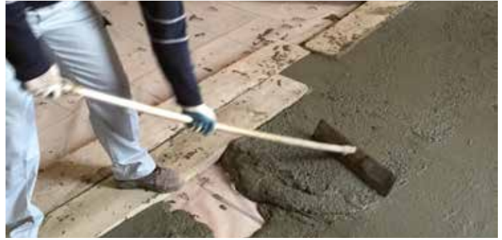
Strengthening of the extrados of a wooden floor
