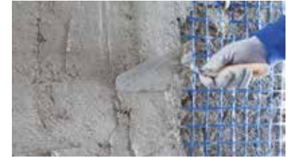
Application of a strengthening package to increase shear-tensile and compressive strength
