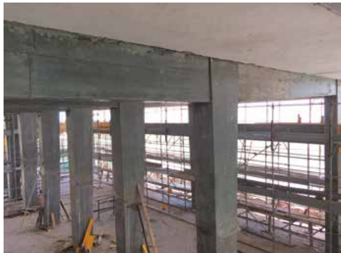
Strengthening of a beam and pillar with a compact jacking
