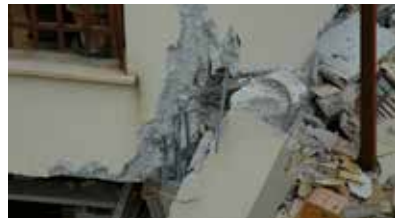
Soft-storey collapse
