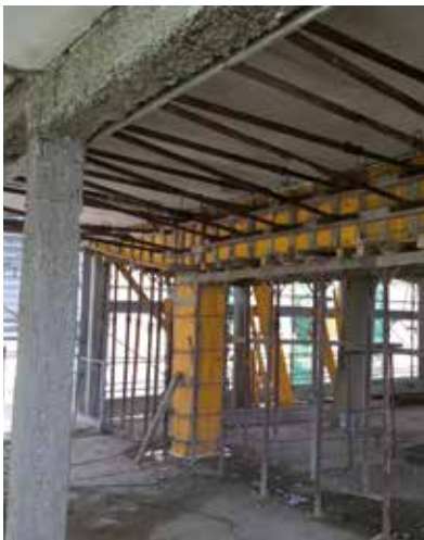
Strengthening of a beam and pillar with a compact jacking
