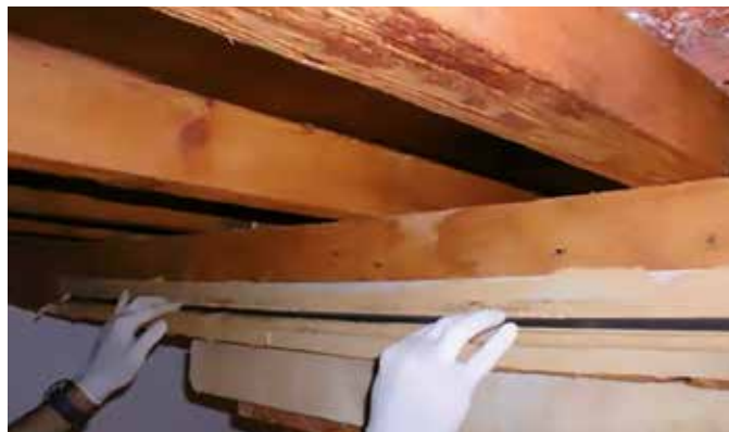
Strengthening of a wooden beam with MAPEROD SYSTEM
