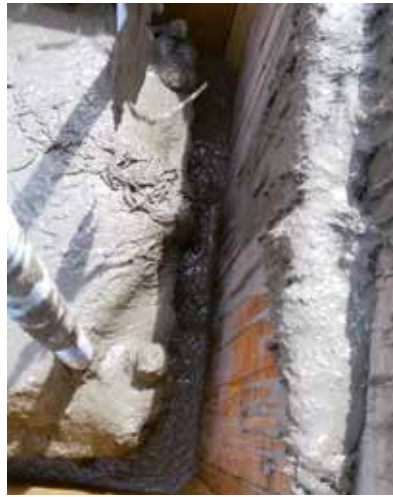
Strengthening of a pillar with a compact jacking
