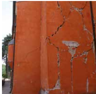
Shear cracks
