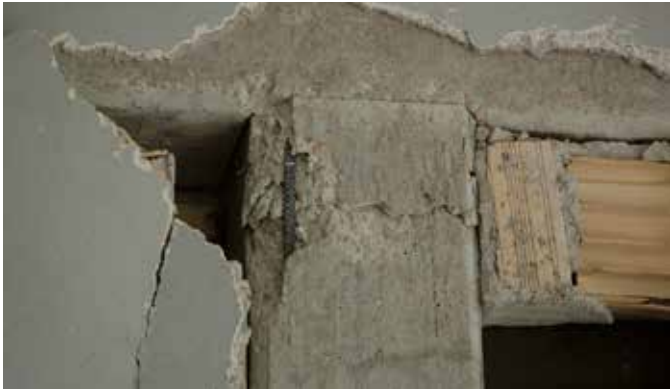
Localised interaction between buffer walls and the reinforced concrete frame
