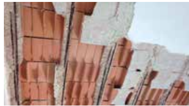
Collapsed floors
