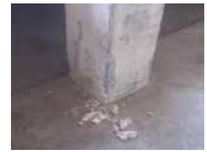
Failure due to combined compressive and bending loads
