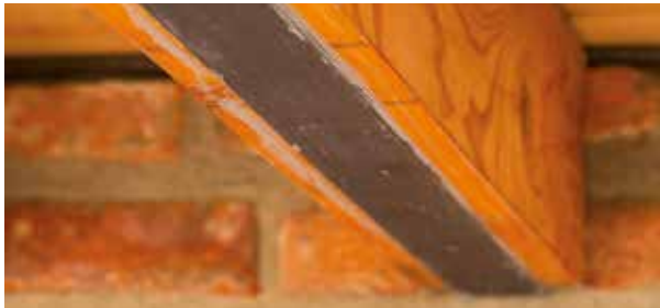
Flexural strengthening of a wooden beam by cladding with CARBOPLATE SYSTEM
