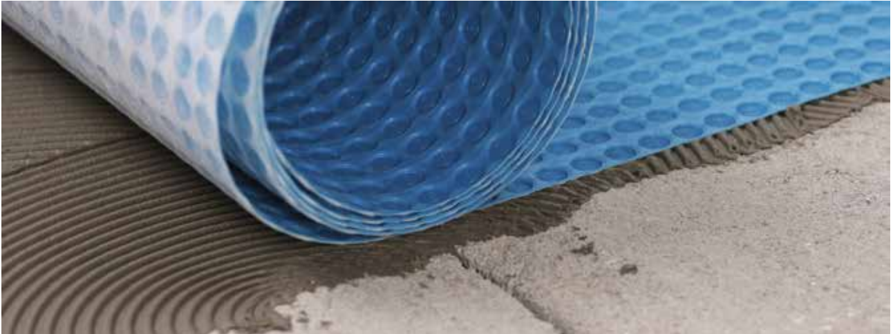
Laying Mapeguard UM 35 on a cementitious screed with control joints.
