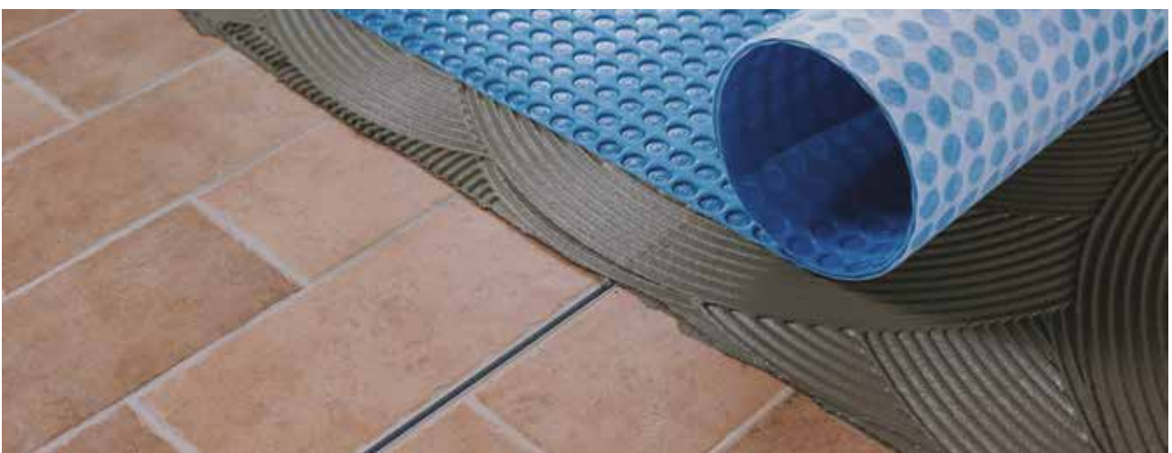
Laying Mapeguard UM 35 on existing ceramic flooring with expansion joints.
