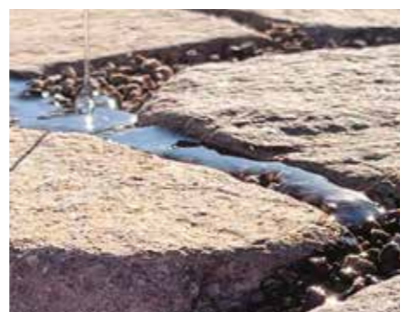
Resin coating grouts with Mapestone Joint Ghost
