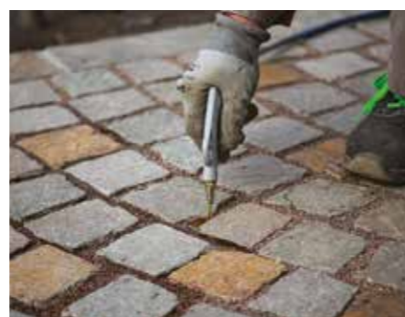
Fill the grouts with Mapestone Joint resin
