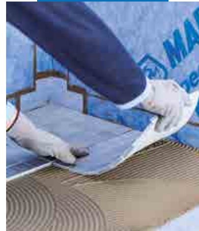
Laying of the tiles
