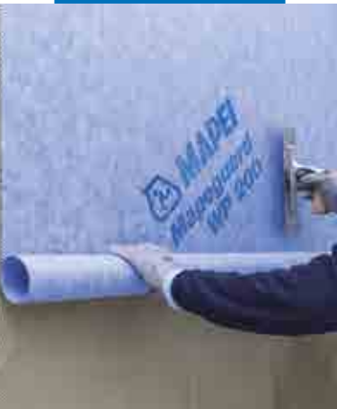
Laying Mapeguard WP 90
