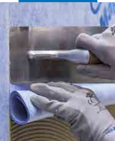
Application of the second sheet
