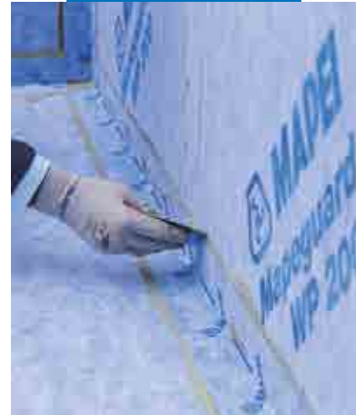
Application of Mapeguard ST
