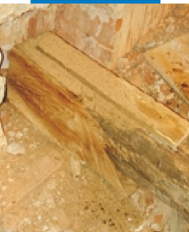
The structural element before applying Mapewood Primer 100
