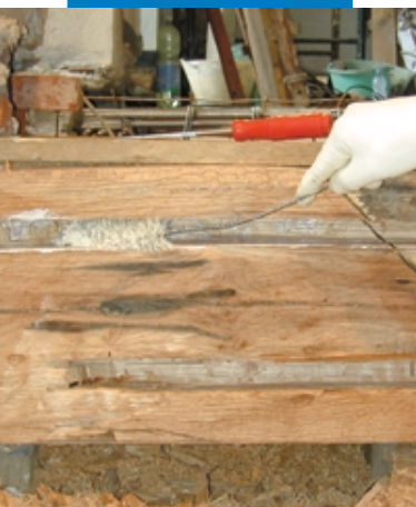
Applying Mapewood Primer 100 with a small bottle brush
