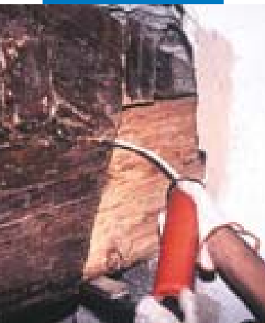
Injecting Mapewood Gel 120
