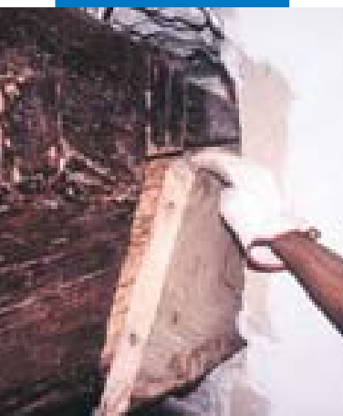
Reprofiling the beam
