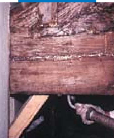
Injecting Mapewood Gel 120
