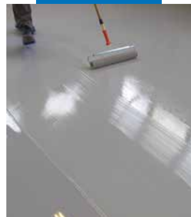
Application of Mapefloor Finish 58 W
