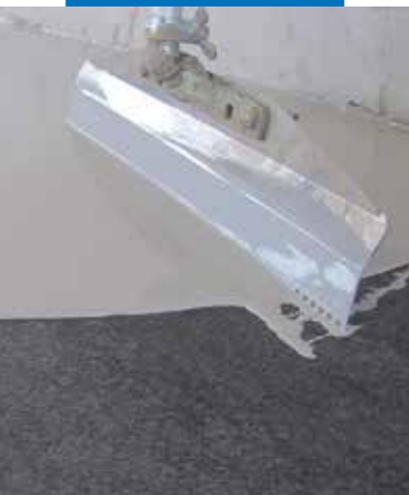
Application of Mapecomfort PU 460 N
