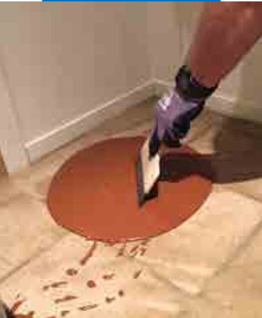
Application of Mapefloor PU 462
