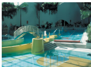
An example of mosaic and klinker installed in a swimming pool
