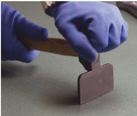
Pressing down the junction between sheets
