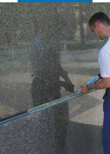
Sealing a façade joint with Mapesil LM
