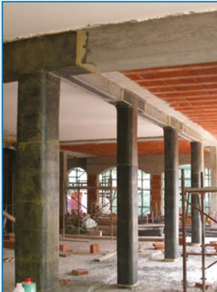
**Joints and pillars strengthened with the MapeWrap C UNI-AX System**
