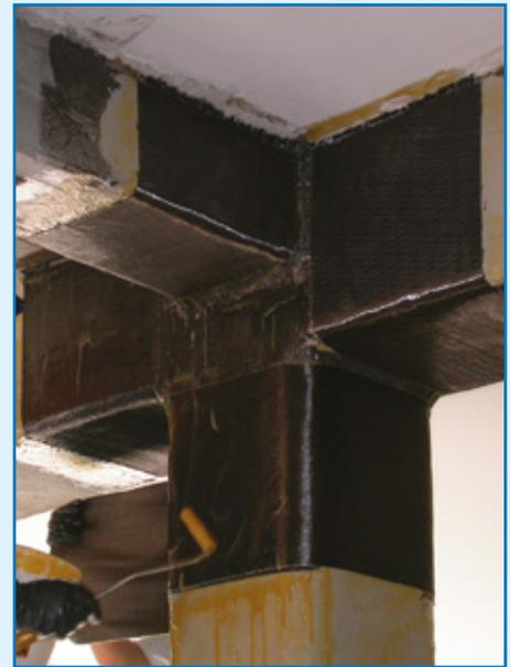
**Beam-pillar joints confined with the MapeWrap C UNI-AX System**
