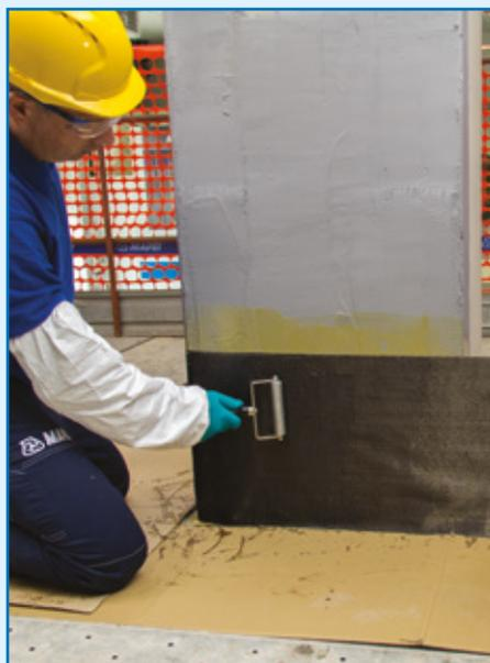
Application of MapeWrap C UNI-AX fibre impregnated with MapeWrap 31
