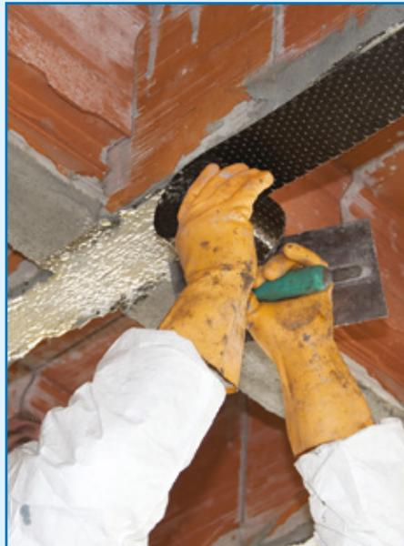
**Flexural strengthening of joists of a brick-concrete floor slab with the MapeWrap C UNI-AX System**
