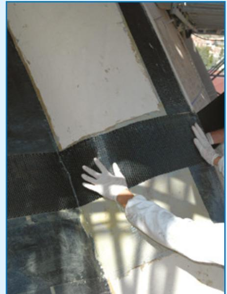
**Domed roof strengthened with the MapeWrap C UNI-AX System**
