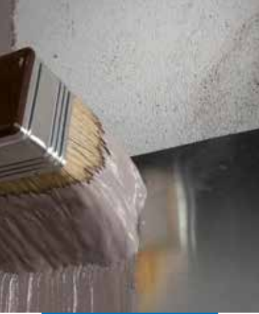
Smoothing over and protecting Mapeshield E 25 with Mapelastic Smart applied with a brush
