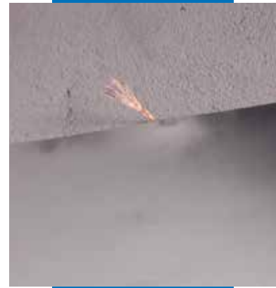
Electric cable previously connected to the reinforcement rods
