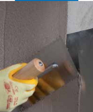
Smoothing over and protecting Mapeshield E 25 with Mapelastic applied with a trowel
