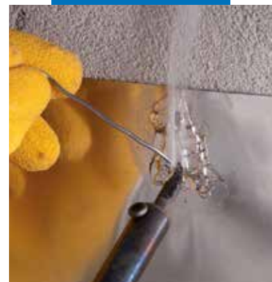
Connecting the electric cable to Mapeshield E 25 by welding
