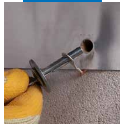
Connecting the electric cable to Mapeshield E 25 with a fastener
