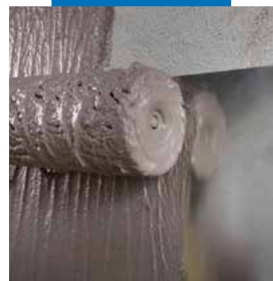
Smoothing over and protecting Mapeshield E 25 with Mapelastik Smart applied with a roller
